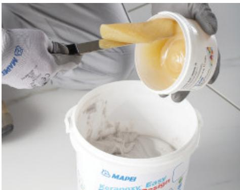
Pour the hardener (component B) in the container of component A
