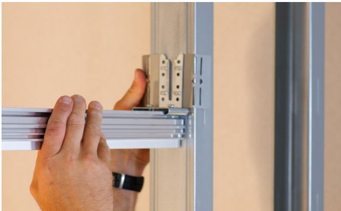
Figure 23: Folding down the lateral flaps
