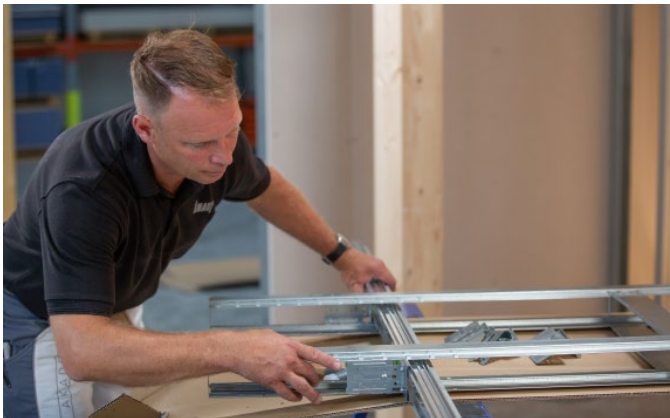
Figure 16: Mounting rail installation
