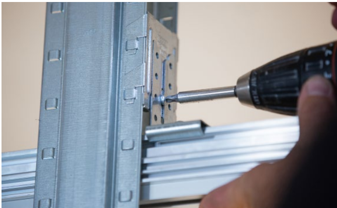
Figure 32: Adjusting the suspension mounting rail
