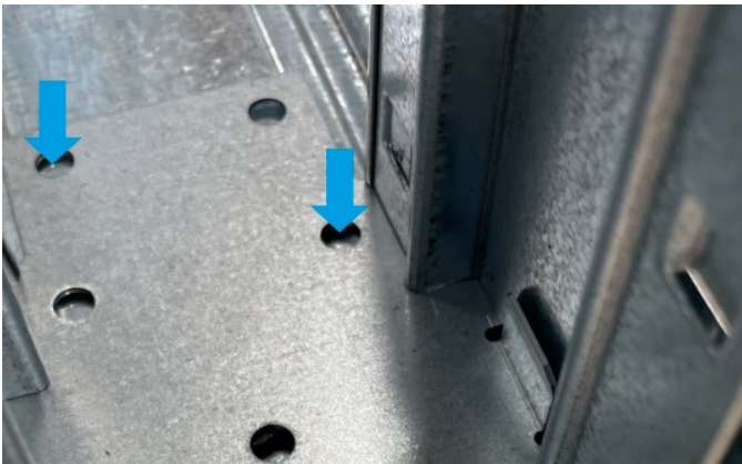
Figure 37: Fasten the connection plates
