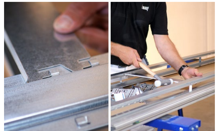
Figure 9: Pre-assemble the pocket
