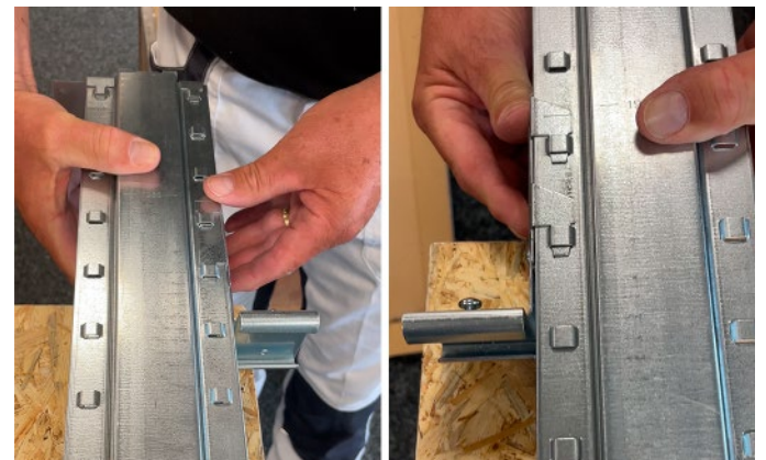
Figure 10: Spacer installation
