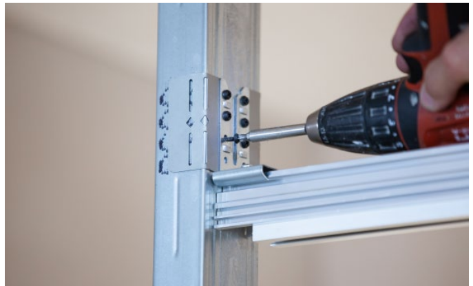
Figure 35: Screw fastening
