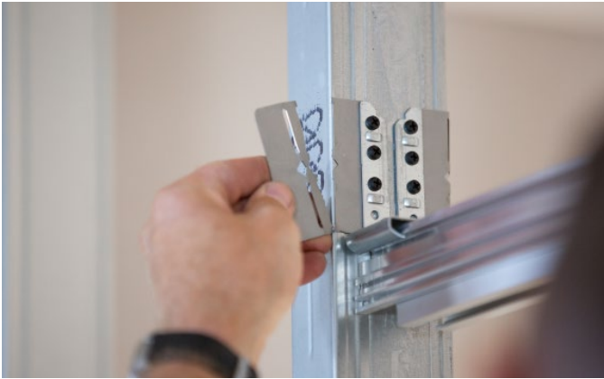
Figure 36: Remove the lateral flaps
