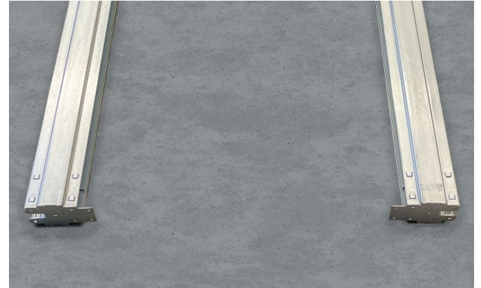
Figure 8: Stud profile alignment
