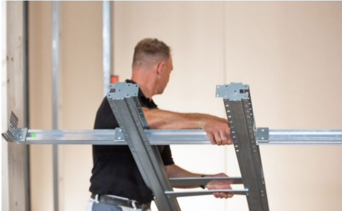
Figure 21: Adjusting the Pocket Kit Easy
