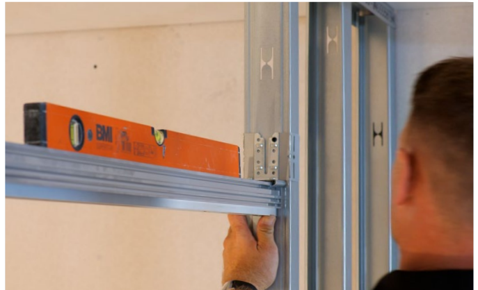
Figure 33: Mounting rail alignment
