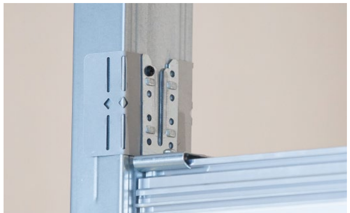
Figure 25: Fixing the suspension
