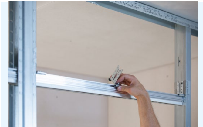
Figure 38: Install the partition frame
