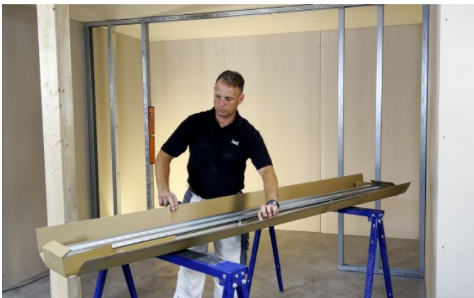
Figure 6: Partly assembled Knauf Pocket Kit Easy (single-leaf – one assembly kit, dual-leaf – two assembly kits)
