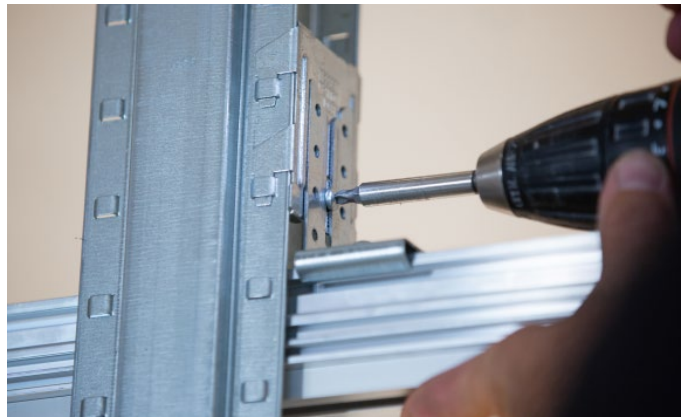
Figure 34: Fixing the suspension mounting rail
