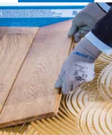
Laying of parquet
