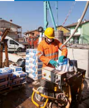
Preparing and pumping the Novoplan Maxi mix using a continuous mixing pump
