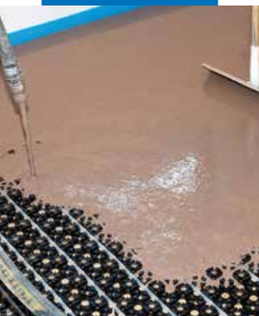
Pumping and levelling off Novoplan Maxi
