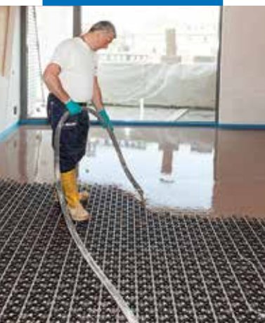
Spreading the mix to completely embed a compact heating system
